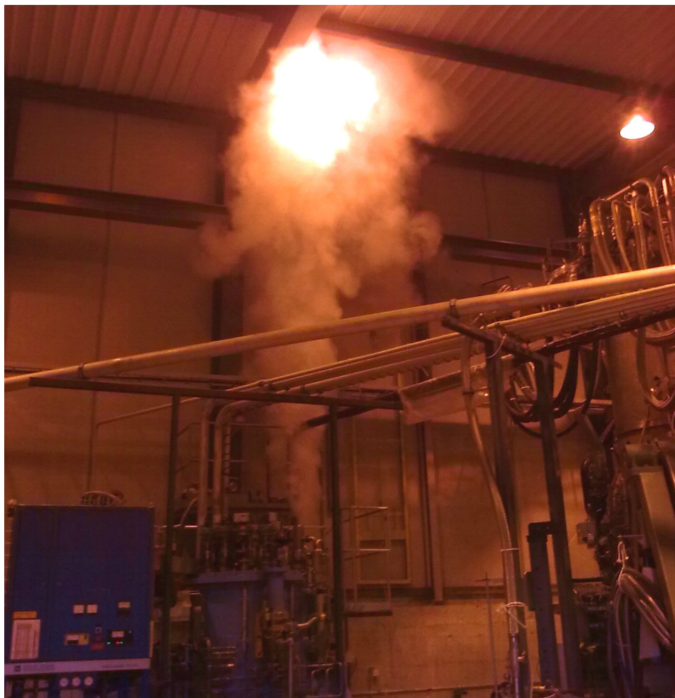
Figure 5-7 Safety release of cryogenic hydrogen during a Magnet Quench in 2010
