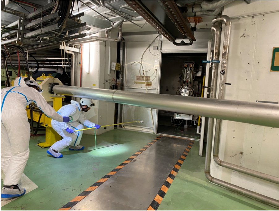
Figure 3.10 Installation of the thermocouples. The long arm used to insert the thermocouple is visible on the photo..
