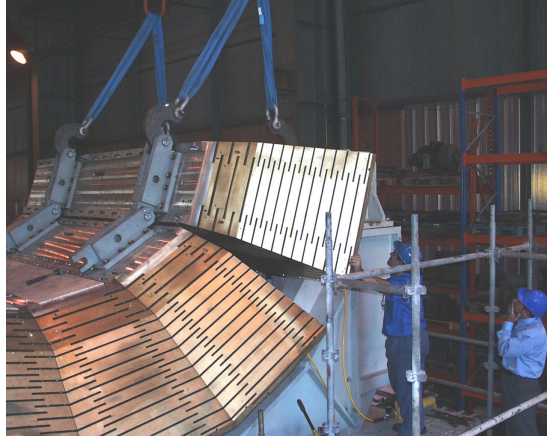
Figure 4.8: The installation of the barrel HCAL wedges, consisting of alternating layers of brass absorber plates and plastic scintillator, each weighing roughly 26 tonnes [27].
