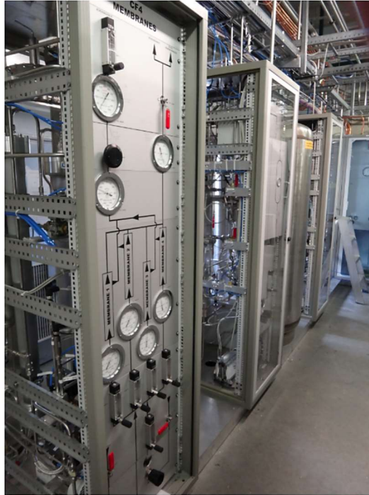
FIGURE 26: Picture of the \text{CF}_4 recuperation plant installed in the surface gas building (SGX5) of the CMS experiment
