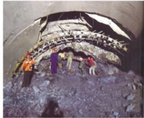
Figure 11: Collapse of the Longxi tunnel during the 2008 Wenchuan earthquake: (left) collapse at the eastern portal of the tunnel, (right) collapse of the lining section at its crossing with a fault [76].
