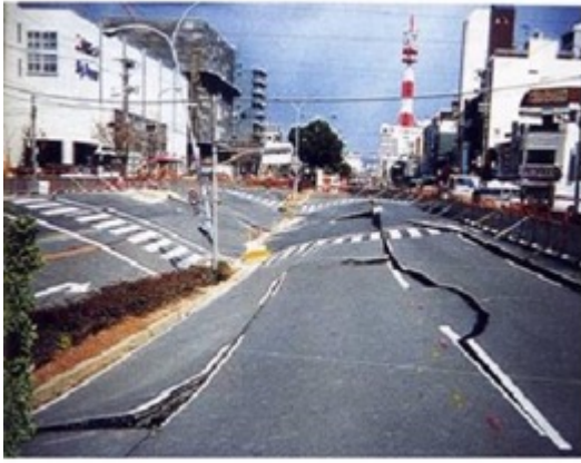
Figure 10: Collapse of the Daikai subway station during the 1995 Kobe earthquake: (left) settlement of the overlaying roadway caused by the subway collapse, (right) collapse of the central columns of the station [76].
