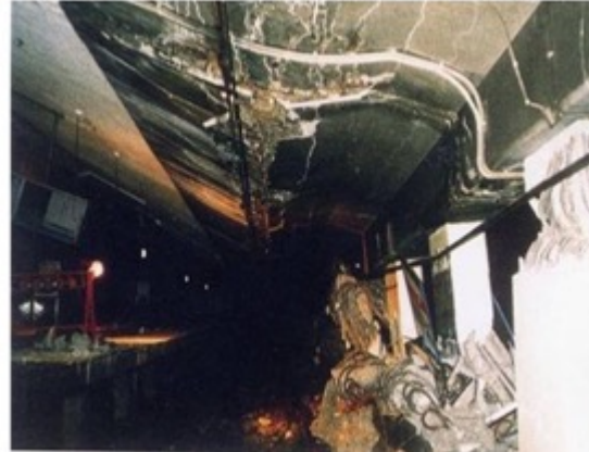
Figure 10: Collapse of the Daikai subway station during the 1995 Kobe earthquake: (left) settlement of the overlaying roadway caused by the subway collapse, (right) collapse of the central columns of the station [76].
