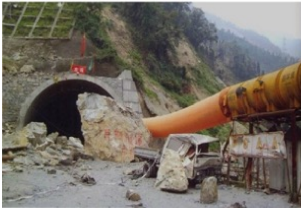
Figure 11: Collapse of the Longxi tunnel during the 2008 Wenchuan earthquake: (left) collapse at the eastern portal of the tunnel, (right) collapse of the lining section at its crossing with a fault [76].
