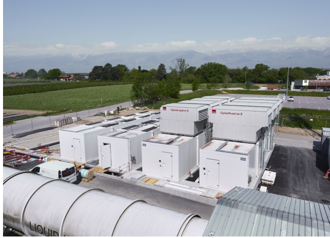
Figure 2.15: The new LHCb containerised data centre under construction at point 8. [58]
