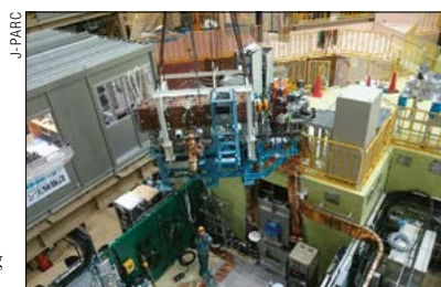
(Left) Installation of the RFQ in the experimental area. (Right) When turning on the RFQ (red), a peak is observed at the expected timing (green). The peak disappears when turning off the RFQ (blue), suggesting acceleration has taken place.
