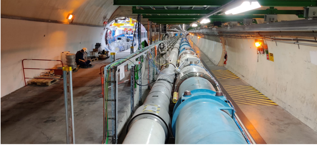
Figure 12.3: Location of the FASER experiment. The experiment is installed inside the side tunnel TI12, formerly used to connect the SPS to the LEP. This tunnel is located on the left side of the picture, right next to the LHC. Later, an additional block of shielding for proton scattered from the LHC beam was added parallel to the LHC right next to the entrance to the TI12. The photograph was taken during the FASER installation in February 2021.
