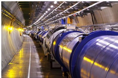
FIGURE 2.1. A view into the tunnel of the LHC.
