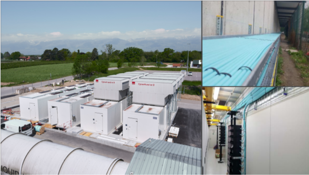
Figure 4.1: New LHCb data centre and the optical fibre cabling to the cavern.
