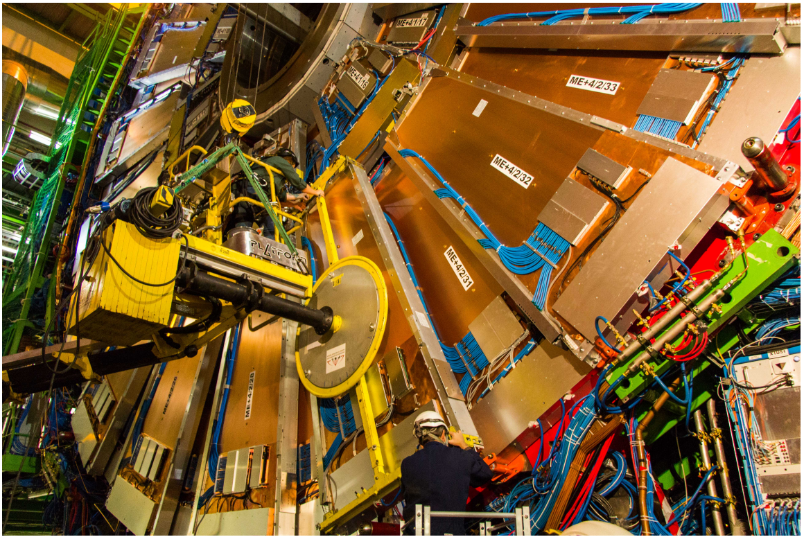
Figure F.3: A closeup of the crane fixture used to install CSCs in the CMS Cavern.
