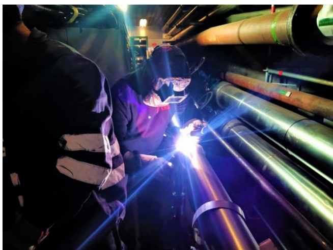
One of the 660 welds already performed in the framework of the Technical Galleries Consolidation Project. (Image: CERN)
