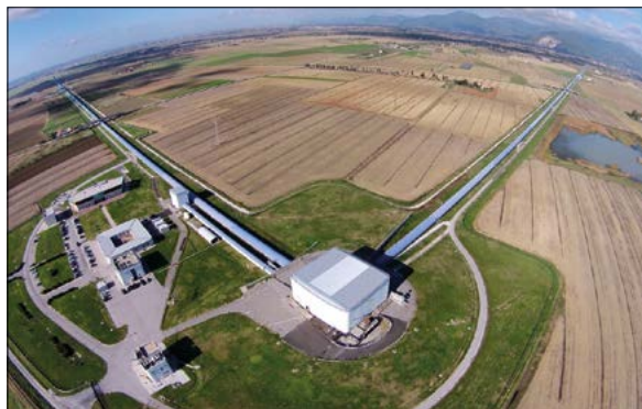
Virgo, located near Pisa in Italy, has arms that are 3 km long and was the first detector in Europe – and the third ever – to register a passing gravitational wave.
