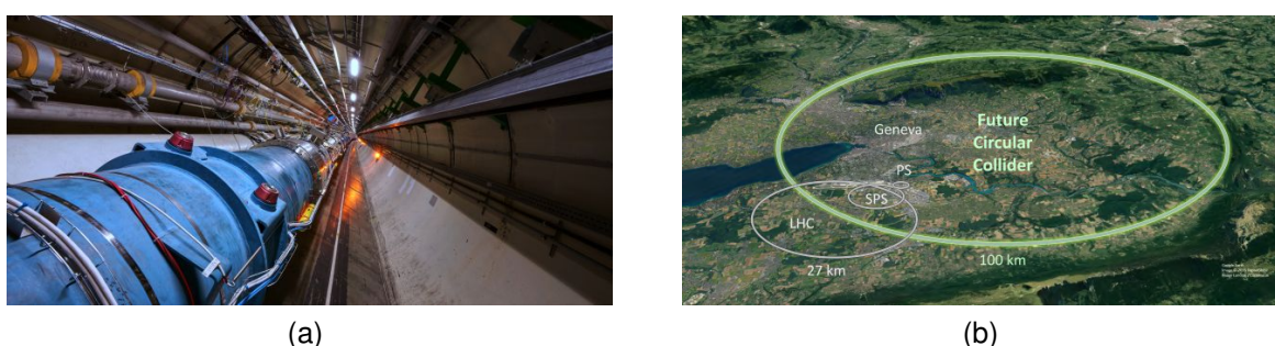
Figure 1.1: CERN accelerator complex; (a) photo of the LHC tunnel with an array of the superconducting magnets (blue); (b) bird's-eye view on the location of the CERN accelerator complex including the PS, SPS and LHC rings. The foreseen location of the 100 km-long Future Circular Collider (FCC) is also indicated [13].
