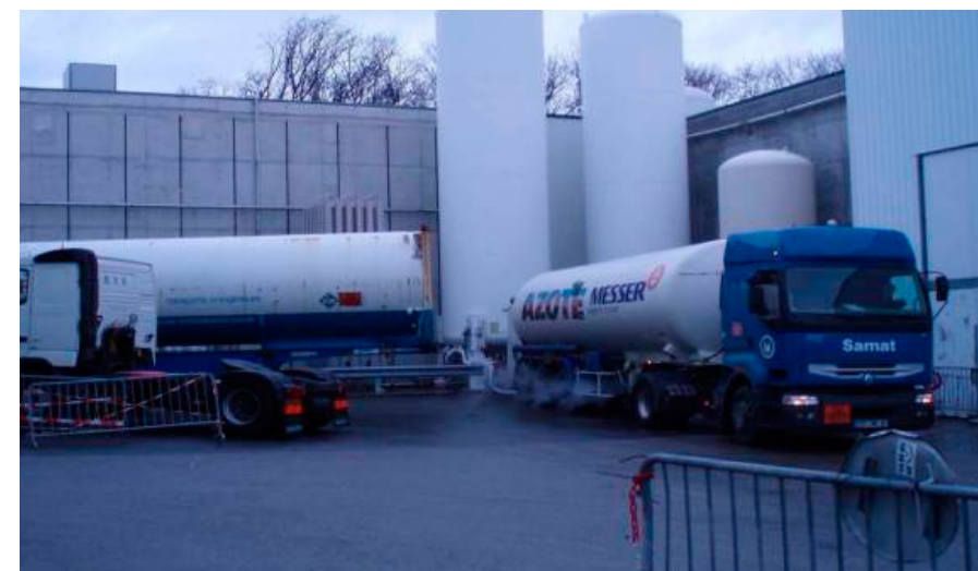
Liquid nitrogen, arriving at CERN on trucks, is injected into exchangers that pre-cool the helium flow used to cool the magnets.
