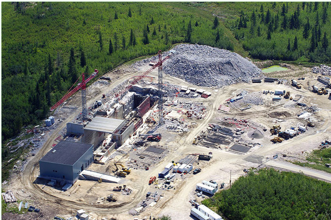
In August 2010, construction crews began installing the roof over the enclosure that will house the NOvA detector. Photo by Dan Traska of Einarson Flying Service.
