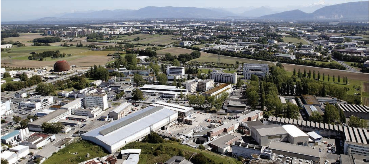
Figure 1.1: CERN photo (site of Meyrin)
