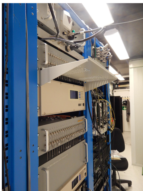
Figure 4.24: The configuration of the laser monitoring system in laser barrack after "Spy-Boxes" installation.
