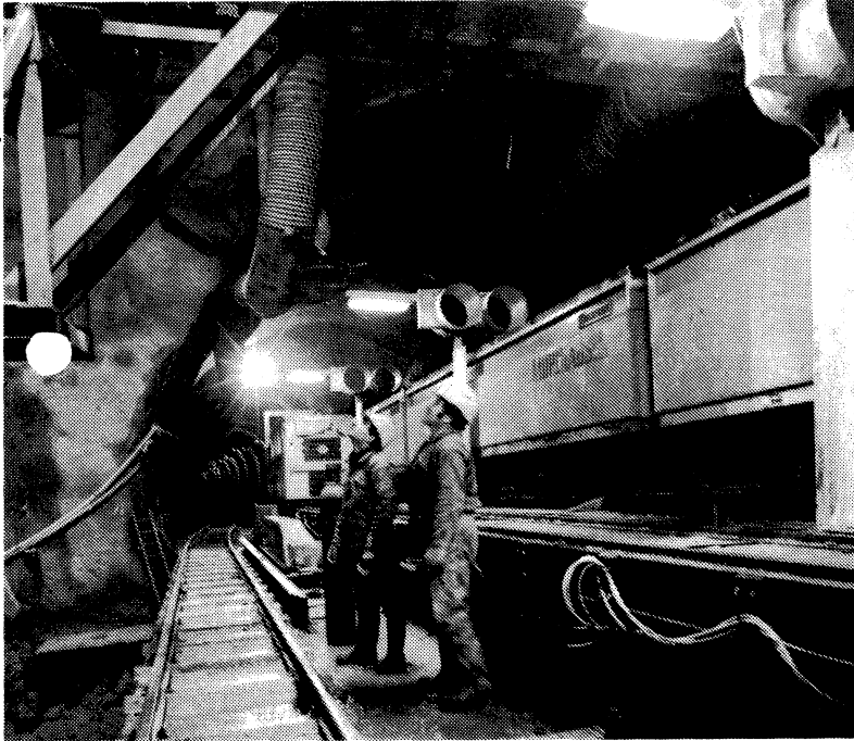
In the LEP tunnel, showing the wagons which remove the soil from the tunnelling machine (Photo 43.3.85)
