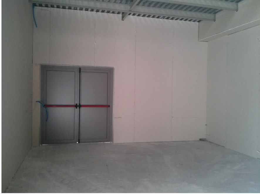
Figure 2.3: The new PL lab in the end of July 2014.
