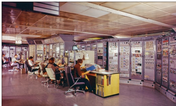
A view of part of the PS control room in 1974, showing rows of individual units with many knobs, switches and oscilloscopes.
