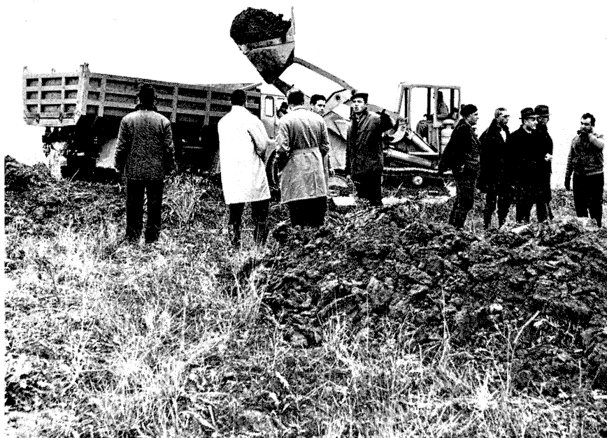
Starting on the ISR tunnel. This photograph was taken on 2 November when work began at the position of the intersecting rings on the French half of the CERN site. The earth excavated in carving out this tunnel, 15 m wide about 7 m high and with an average diameter of 300 m, will be transported to a dump on the opposite side of the Geneva - St-Genis road using a tunnel cut under the road. The earth required later as shielding around the storage rings will be stocked on the site.
