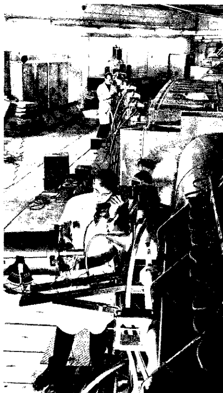
A photograph taken in the synchrotron ring tunnel at the point (straight section 74) where the fast ejected proton beam is taken out for the neutrino beam-line. The proton beam passes through the tunnel wall (top centre) and is directed onto a target. The positive pions and kaons produced in the high energy collisions are converged by magnetic lenses towards the heavy liquid bubble chamber. They decay after a very short time producing the required neutrino beam.
