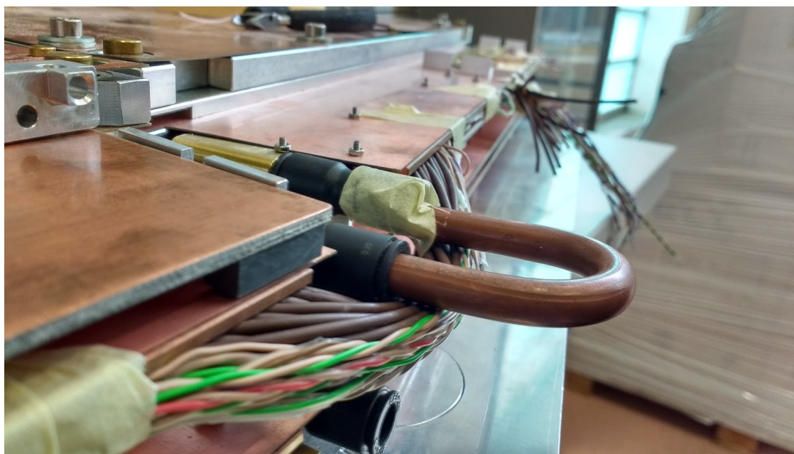
Figure 3.13: NSW Micromegas mockup of SM1 and SM2 in 2016 during an effort to emulate the final routed services, which at the time were out of defined envelopes.
