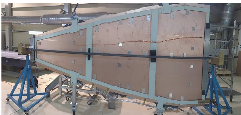
Figure 3.37: MDM modules installed on NSW spokes.
