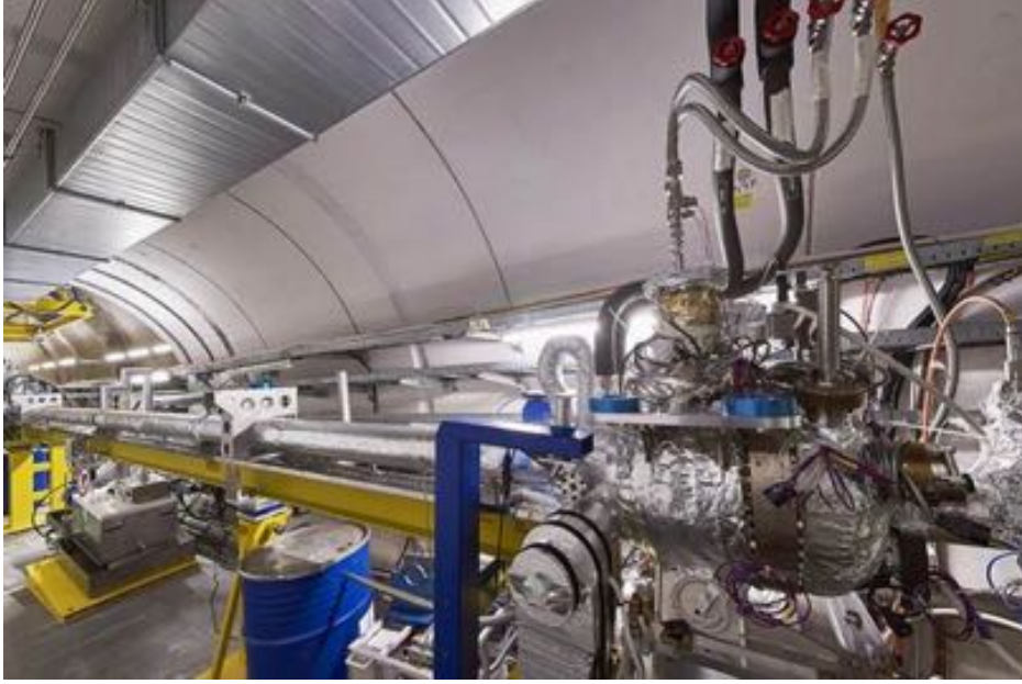
Figure 1.3: Photograph of the rubidium vapor source installed in AWAKE.
