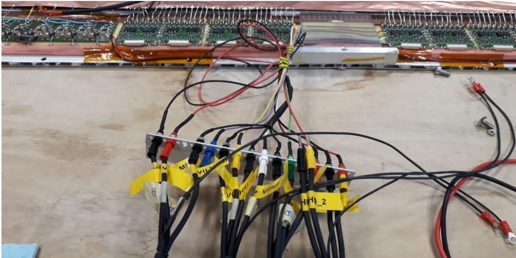
Figure 3.10. The patch-panel with the labeled 6 adjustable low voltages (LV) cables for the the powering of the front-end FEBs: V_{TH} , V_{DIS} , V_{AMP} , V_{PU} , V_{LVDS} , V_{PREAMP\_Left} , V_{PREAMP\_Right}
