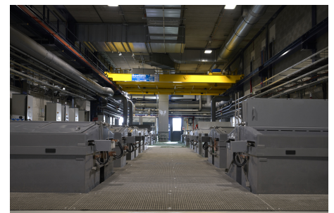
One of the laboratories for the surface treatment of vacuum equipment of the Building 107. The tanks with a double skin are installed above high-tech retention basins with a special coating to withstand chemicals. (Image: Maximilien Brice/CERN)
