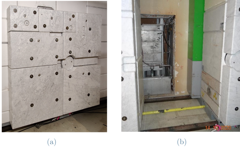
Figure 2.6: The mobile shielding: (a) in the closed position (b) in the open position [25].
