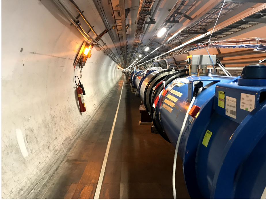
Figure 2.1: The LHC tunnel. The blue cylindrical structures contain the superconducting dipole magnets that bend the particle beams circulating inside the LHC. (September 2019, photo credits: MGF)
