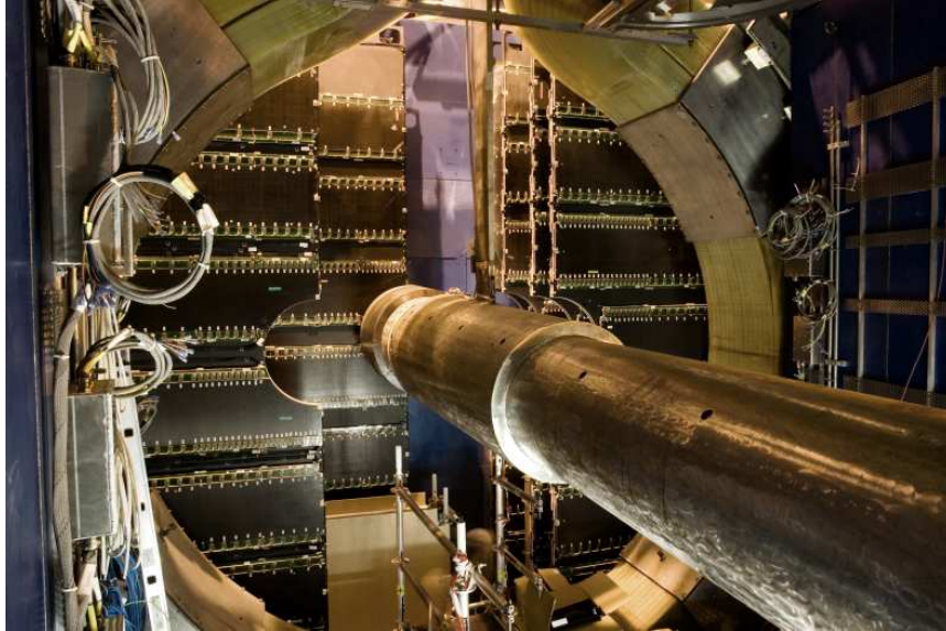
Figure 2.10: Layout of the tracking Stations 4 and 5, installed in the ALICE cavern.
