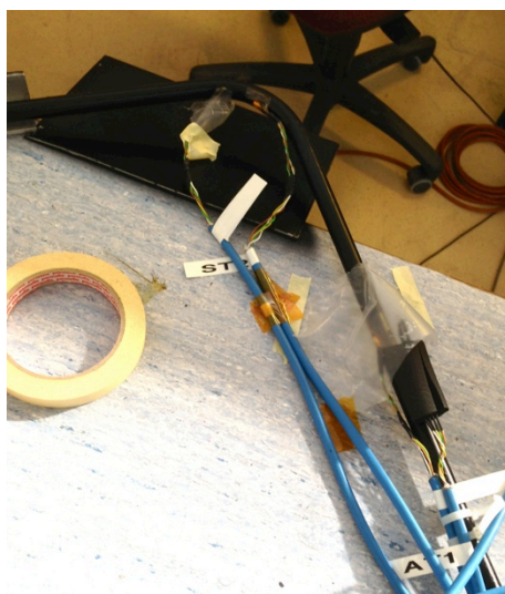
Figure 6-24 Temperature sensors installed on the bent rigid part of the transfer line
