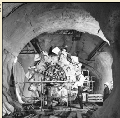
The mole being installed underground at the point where boring is beginning. Its 7 km journey around the ring is expected to be completed by autumn 1974. The machine, 80 m in length, comprises the 4.8 m diameter head, shown here, pressure and supporting pads, an operator's cabin, electrical equipment, conveyor belts, tunnel-lining system, skip changer and spoil-removal train.
