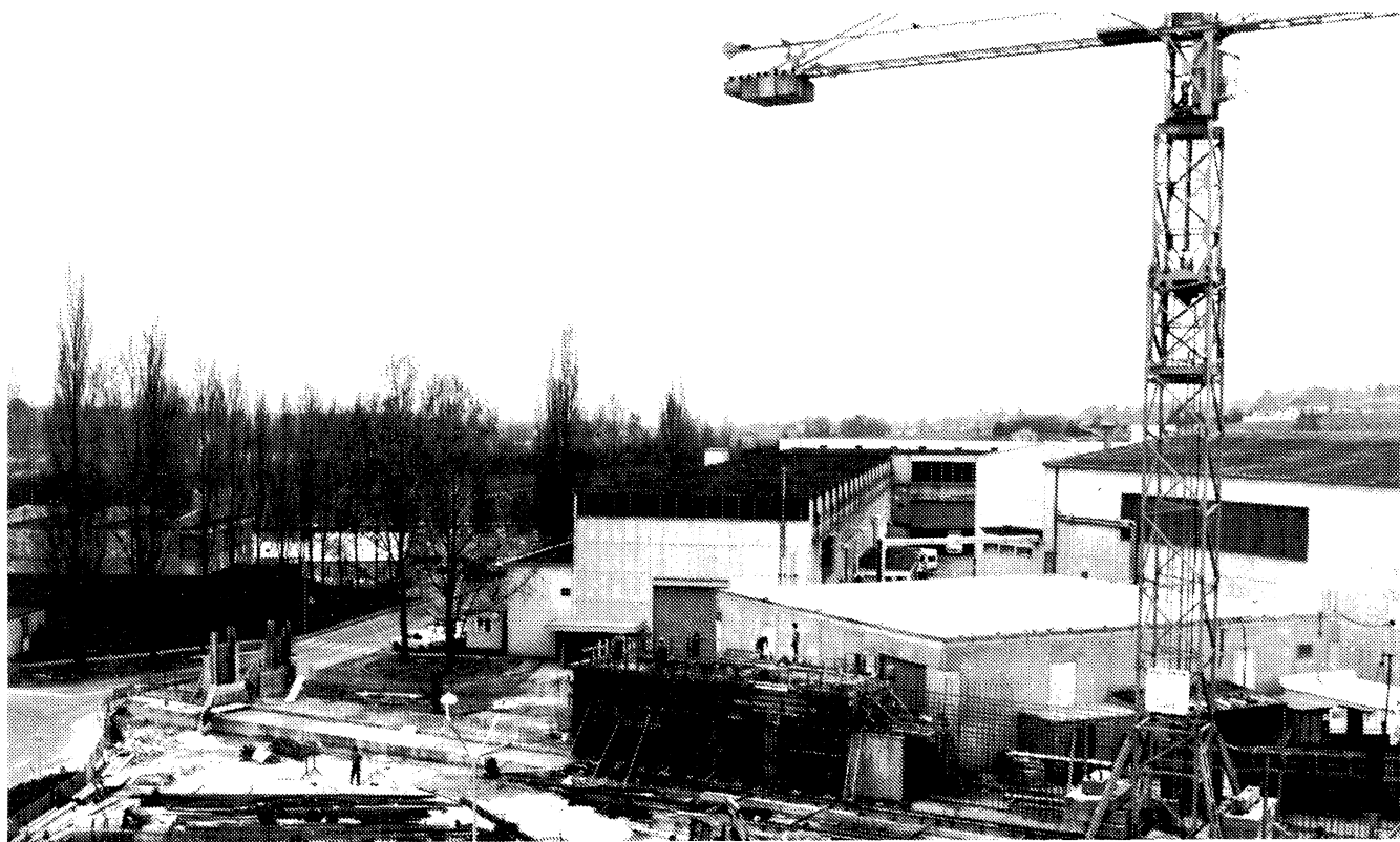
The tunnel for the LEP Injector Linacs (LIL) takes shape near the PS.
