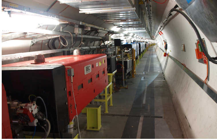
Figure 11: Photo of the proton transfer line from the SPS to AWAKE.
