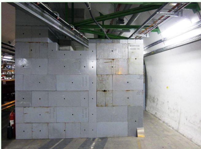
Installation of shielding at Point 1.
