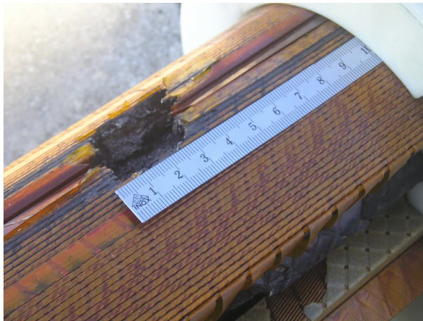
Figure 5.22: Coil damage due to a inter-turn short in a LHC pre-series dipole.
