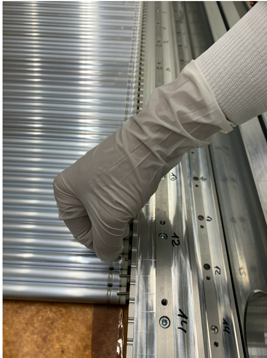
(a) Placing the grounding screws.
