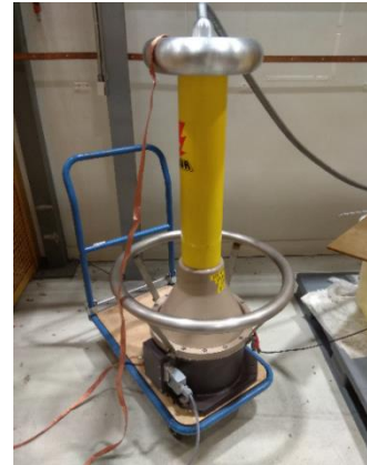
Fig. 34. The High Voltage unit
