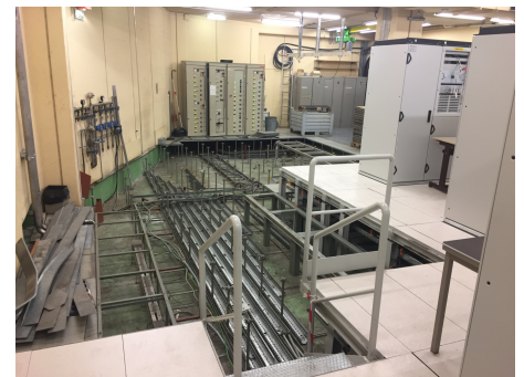
The room housing the power converters and the control system for the PS Booster is completely empty during LS2. All cables running under the false floor are removed before installing the new power and control system (Image: Matthias Haase/CERN)
