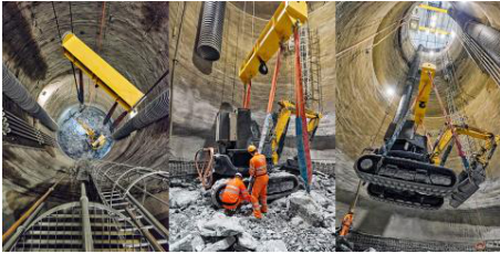
A montage of three photos showing an excavator in one of the two shafts that were dug for the High-Luminosity LHC (Images: Antonino Panté*)
