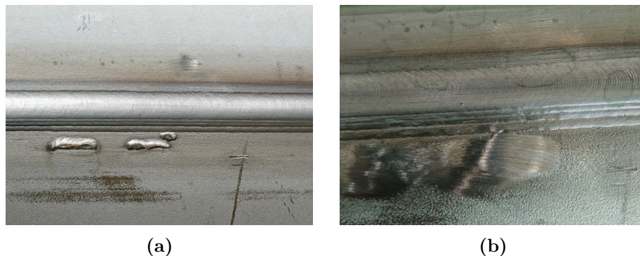
Figure 3.13: (a) Surface features from the weld procedure. (b) Grinded tack weld and pressure mark.
