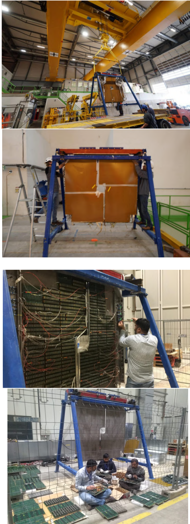
FIGURE C.2: Dismantling PMD at the surface area: (from top to bottom) PMD moved from cavern to surface area by crane, PMD is placed at the surface area (radiation protected zone) with the help of a support structure (blue frame), electrical cables and gas flow tubes removal and finally module wise dismantling.
