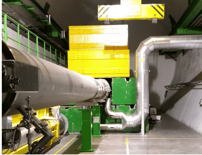
Figure 2.5: Picture showing the dump block within its shielding and the connecting line connected to it, from [15].
