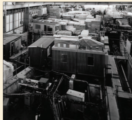
In the East Hall looking towards the PS. Wooden huts house the small computers being used on-line in electronics experiments clustered around the slow ejected beam. From the April cover (below).
