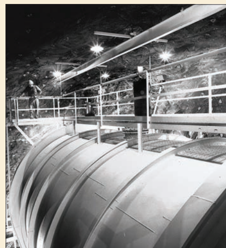
One end of the huge tank of tetrachloroethylene catching neutrinos down a South Dakota gold mine. (Image credit: BNL.)
